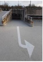
drainage pipes/gullies were installed to the base of the ramps. The entire top deck coating of each carpark was removed, hybrid galvanic anodes were installed to each area where high chlorides had been identified, and the deck surfaces were coated with a Tremco MMA Flexible Waterproof System. The perimeter gutter system of the office buildings were re-lined with a liquid applied waterproof system and expansion joints and plasterboard ceilings were replaced.
